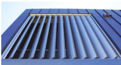
EX-6 ADJUSTABLE VERTICAL ALUMINUM LOUVERS
